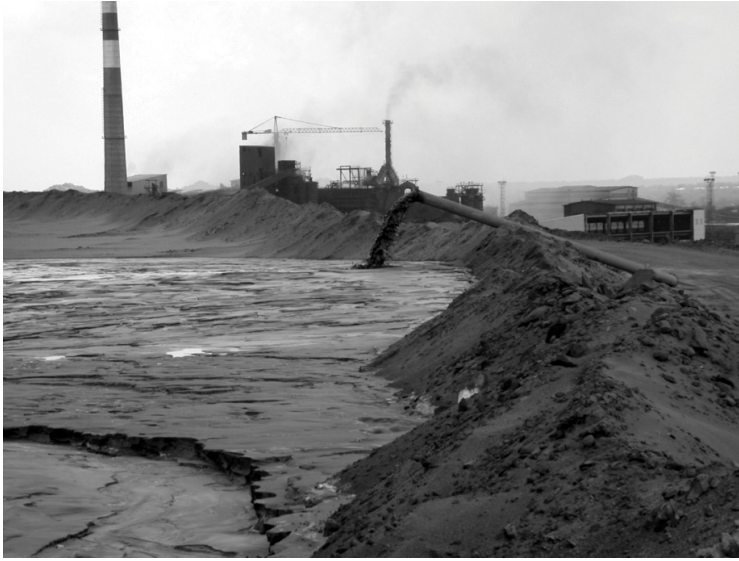
Figure 10.1 Depositing sulfidic mine tailings as slurry on top of the tailings dump (ore processing plant in the background).
